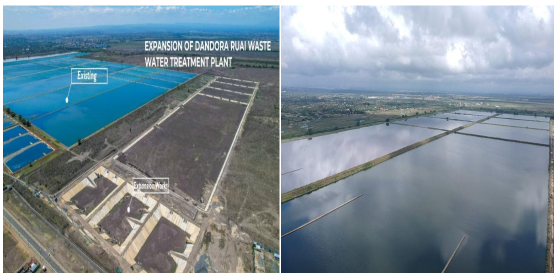
Dandora Estate Sewerage Treatment Plant features the largest wastewater stabilisation pond in Africa, treating 80,000 m 3 of sewerage per day (80% of Nairobi's wastewater).
