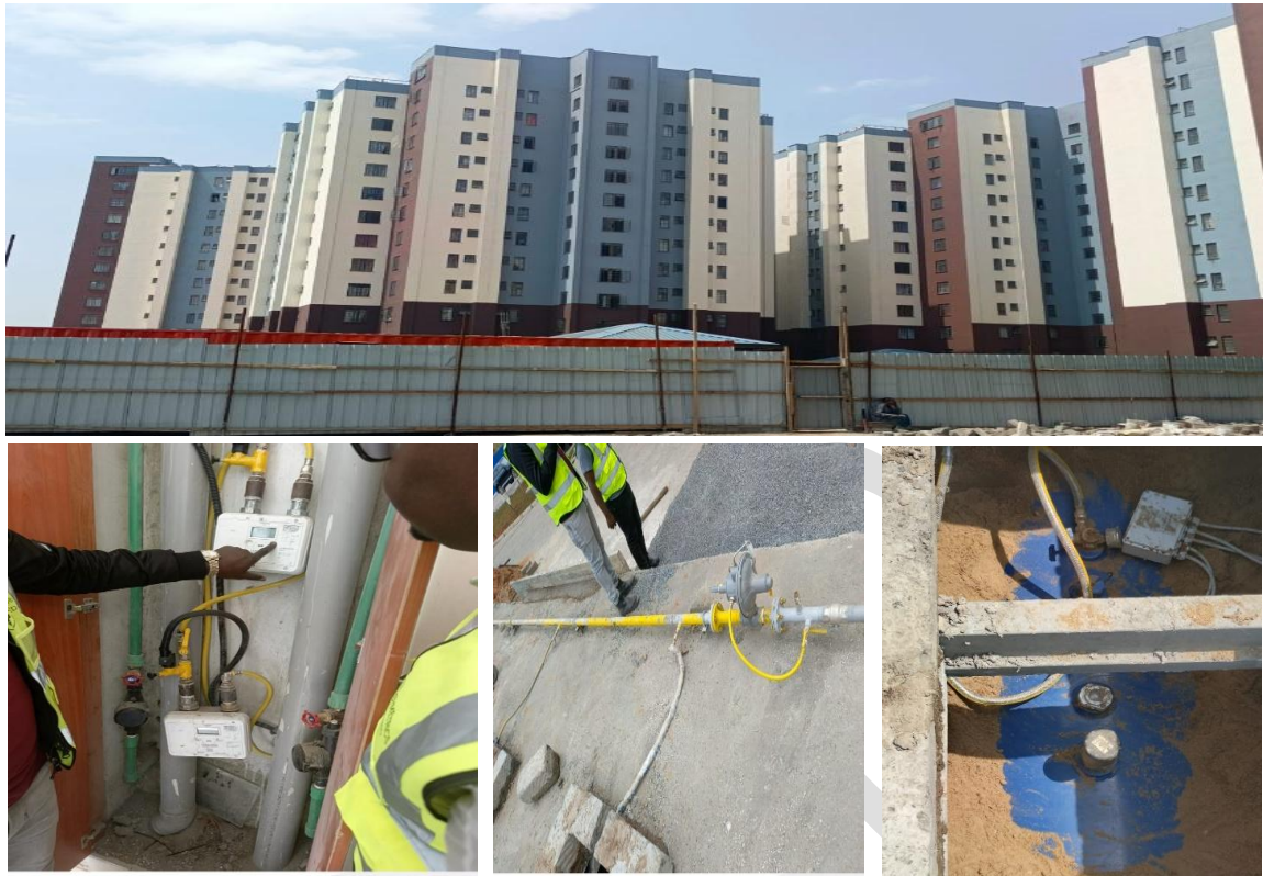
LPG Reticulation Infrastructure installed at Mukuru Affordable Housing
