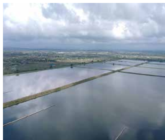
Dandora Estate Sewerage Treatment Plant features the largest wastewater stabilization pond in Africa, treating 80,000 m 3 of sewerage per day (80% of Nairobi's wastewater)
