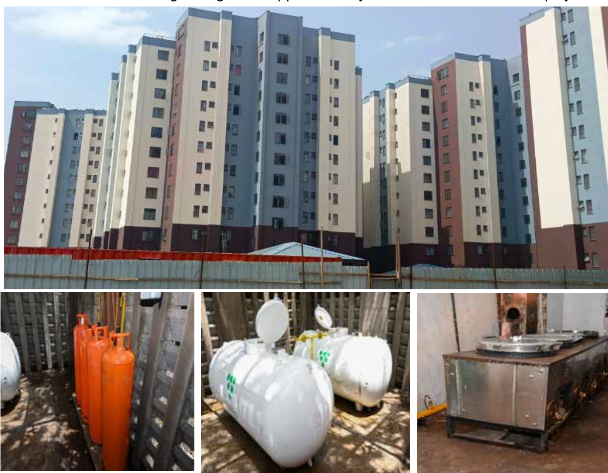
LPG Reticulation Infrastructure installed at Mukuru Affordable Housing
